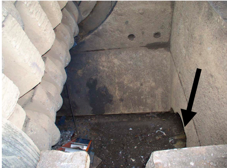
Figure 5. View into shredder box from platform outside of box showing access point from outside conveyor
